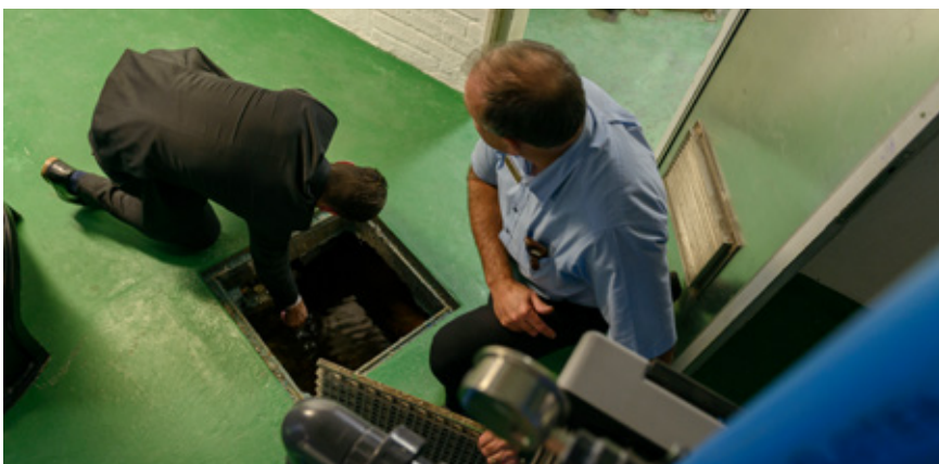
Chief Engineer Andrew Gartshore (right) at The Westin Cape Town shows the sea water that was previously pumped out of the hotel basement.
