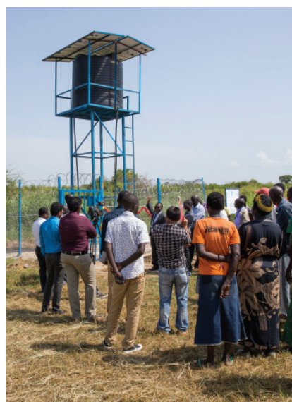
UN Mission in South Sudan hands over solar-powered water facility to Gormoyok Village
