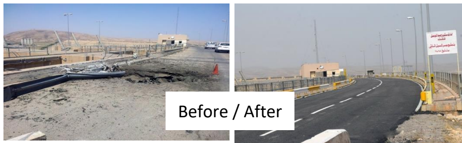
Figure 3. Mosul dam spillway bridge before and after the emergency rehabilitation.
