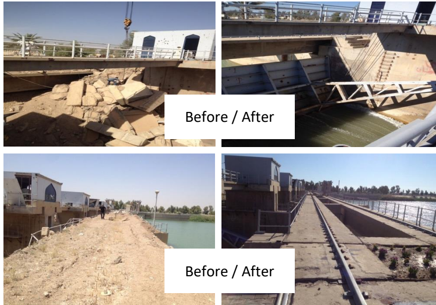
Figure 4. Fallujah barrage before and after the emergency rehabilitation.
