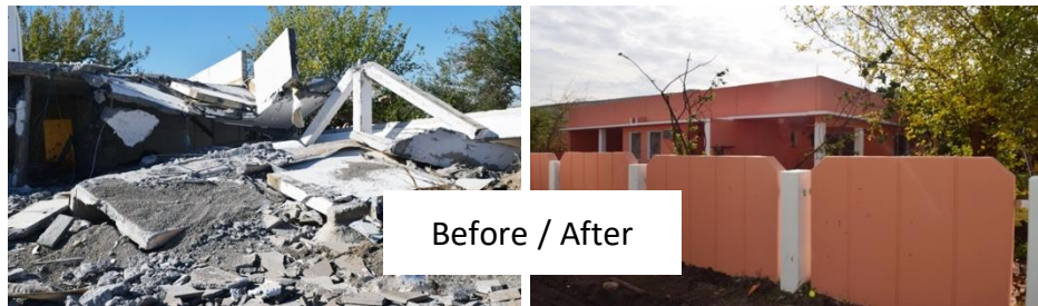
Figure 2. the Mosul dam housing camp before and after the emergency rehabilitation.
