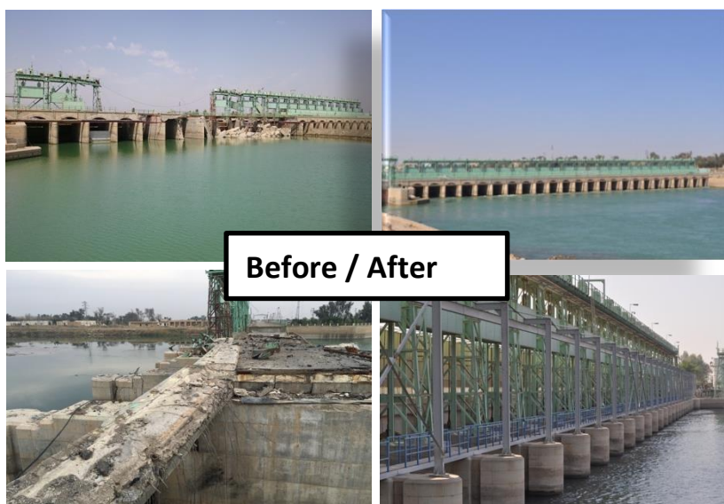
Figure 5. Ramadi barrage before and after the emergency rehabilitation.
