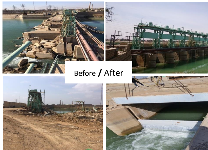
Figure 6. Al-Warar barrage before and after the emergency rehabilitation.
