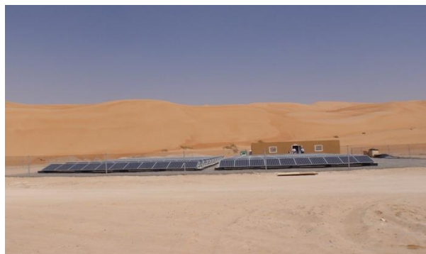
Figure 30: Small scale solar powered RO desalination plant in Abu Dhabi.
