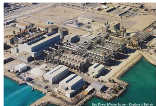
Figure 10. Desalination Plant in Bahrain
